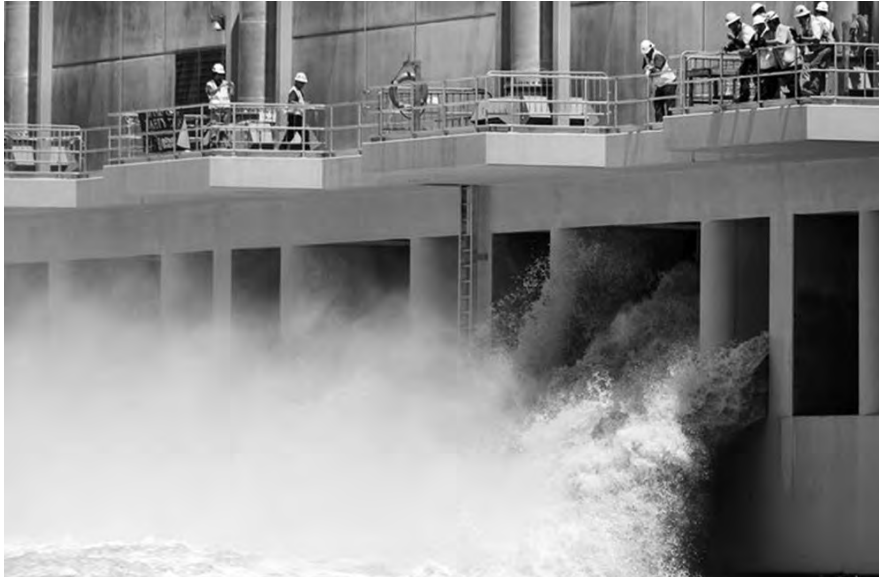
The West Closure Complex Pump Station in New Orleans, Louisiana—designed by ARCADIS, it is the world's largest stormwater pump station, capable of pumping nearly 20,000 cubic feet of water per second out of inhabited areas of New Orleans and into the Gulf of Mexico. photo credit: ARCADIS
