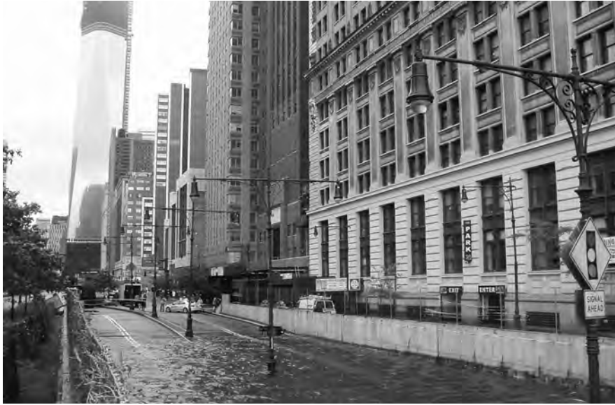
Flooding of the Brooklyn Battery Tunnel, looking northward toward the unfinished Freedom Tower photo credit: ARCADIS
