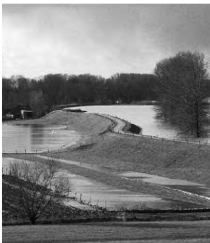
Reclaiming and protecting marshy land was and is a communal enterprise that people have to do together.
