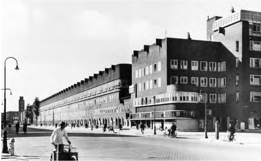
Contemporary streetview of the Hoofdweg in the direction of the Mercatorplein, classic Amsterdam School architecture by H.Th Wijdeveld (1885-1987), editor of the renowned avant-garde journal Wendingen .
