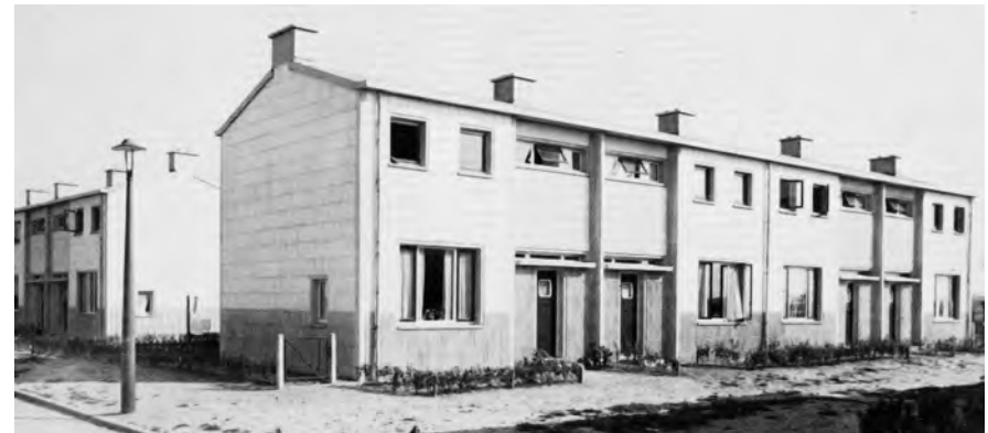
Early example of the Dutch 'doorzonwoning', or mass produced, row houses in the village of Rheden, 1949, designed by the Rotterdam architect Willem van Tijen (1894-1974).
